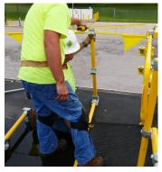
**5.** When placing the post/outrigger assemblies, ensure that the bottom surface of the slipper and the roofs make full contact with the supporting surface. The heel of the slipper in each post/outrigger assembly should bear against the roof parapet. If the parapet is absent, the heel of the Slipper must be a minimum of 12" from the roof edge.
