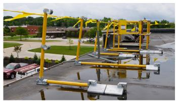
**7.** Install 20 ft sections of 1.9" OD FRP tube top and mid rails through the open cross over fittings on the posts. Torque the set screw to 7.5 lb-ft (10.1 N-m). Add thread locking compound to the set screws to prevent loosening. Splice the rails together using PN 504701 Rail splice assembly which consists of two PN 793149 Sleeve joints.
