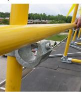
**8.** At returns (unsupported terminations of the guardrail), connect the two ends of the 1.9" OD FRP tube using PN 5045010 Return Assembly which consists of a length of 1.9" OD FRP tube and two PN 793125 Two Way Elbows. Torque set screws to 7.5 lb-ft (10.1 N-m). Add thread locking compound to the set screws to prevent loosening.
